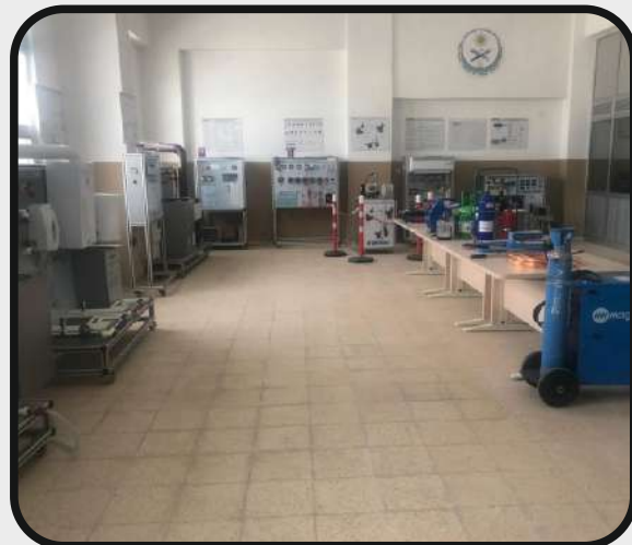
SIMAV VOCATIONAL AND TECHNICAL ANATOLIA HIGH SCHOOL INSTALLATION TECHNOLOGY AND AIR CONDITIONING WORKSHOP
